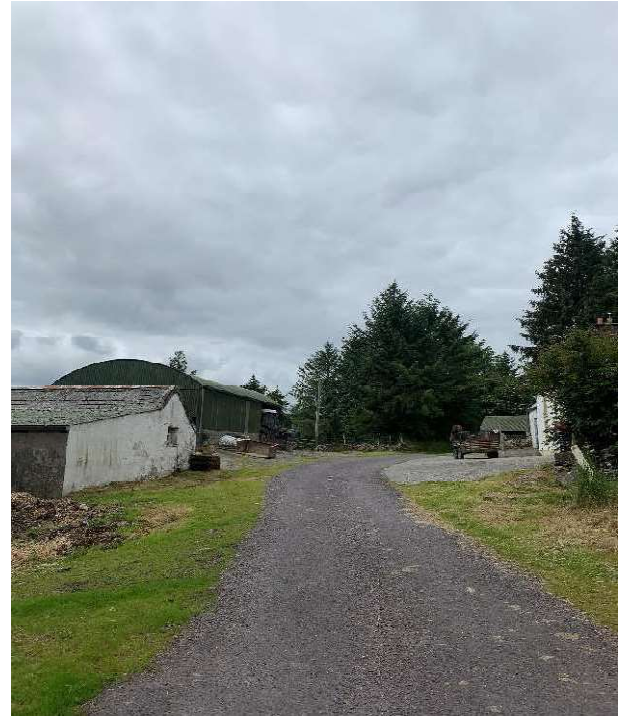
Image : 56 Existing farm buildings on both sides of the road at this location
