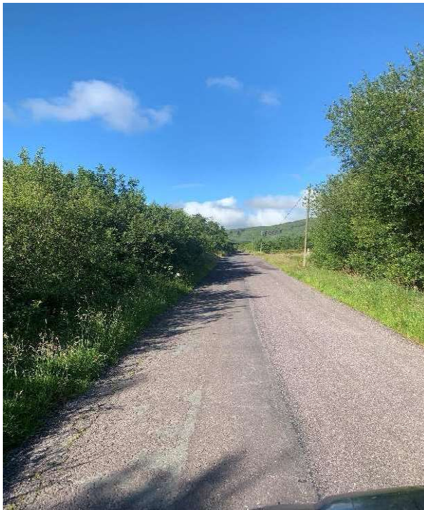
Image : 3 Existing cable running down road
