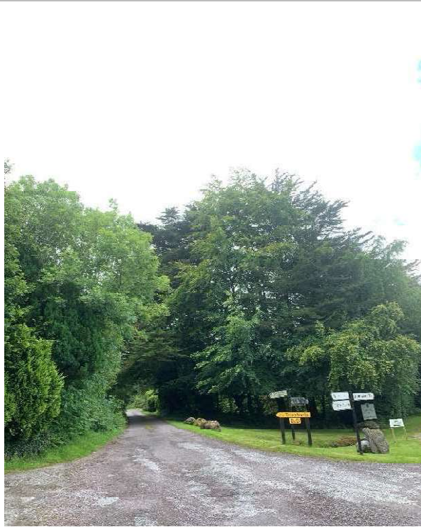
Image : 43 Road goes from double carriageway to single as proposed cable route deviates to the right
