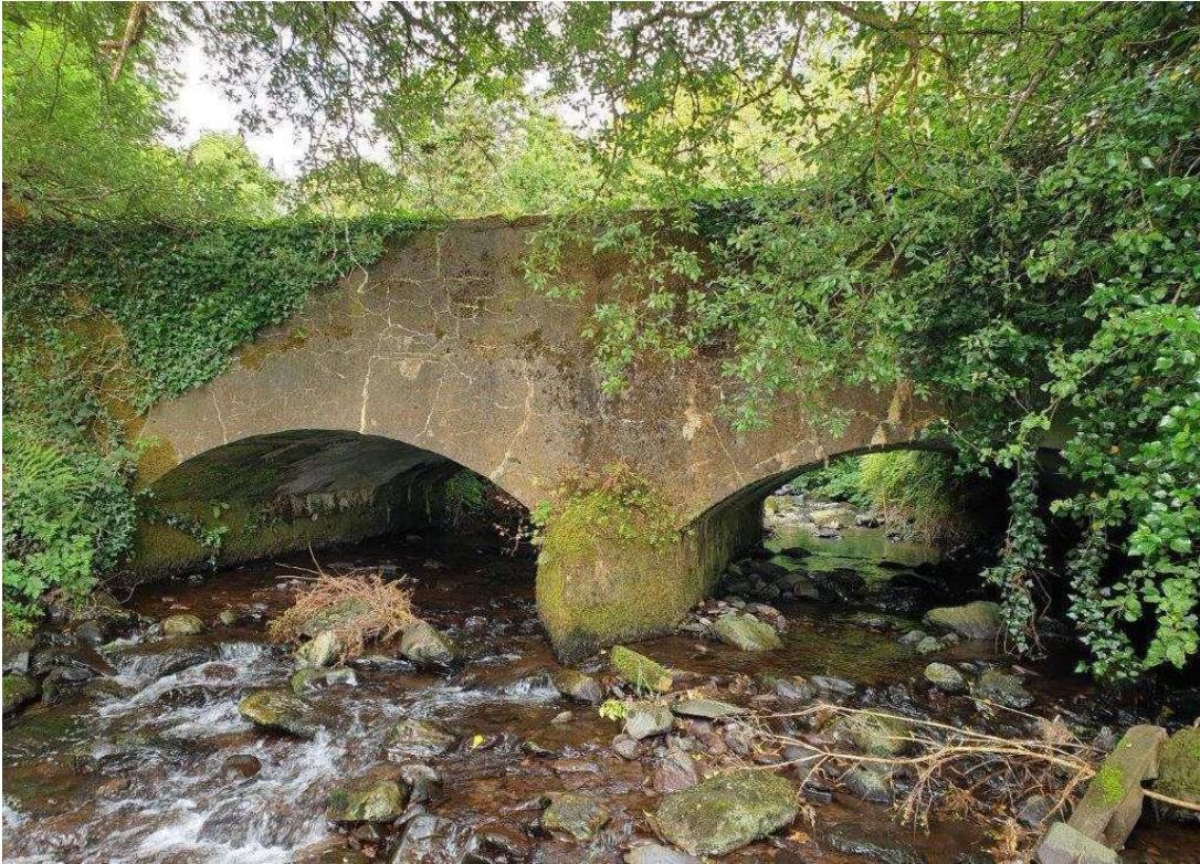
General view of south elevation
