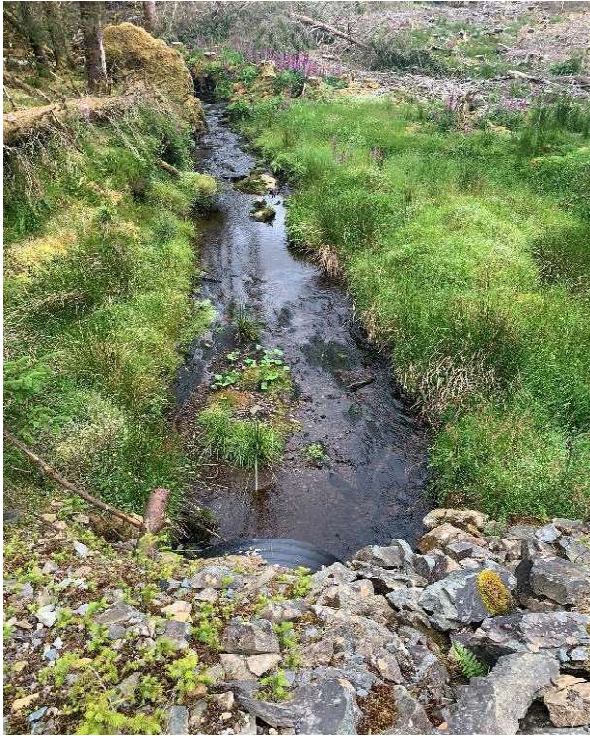
Image : 82 Stream crossing track at this location with a partial collapsed storm pipe
