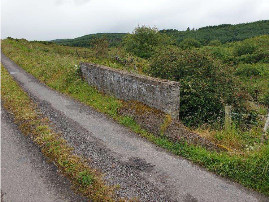
General view of bridge surface and west parapet
