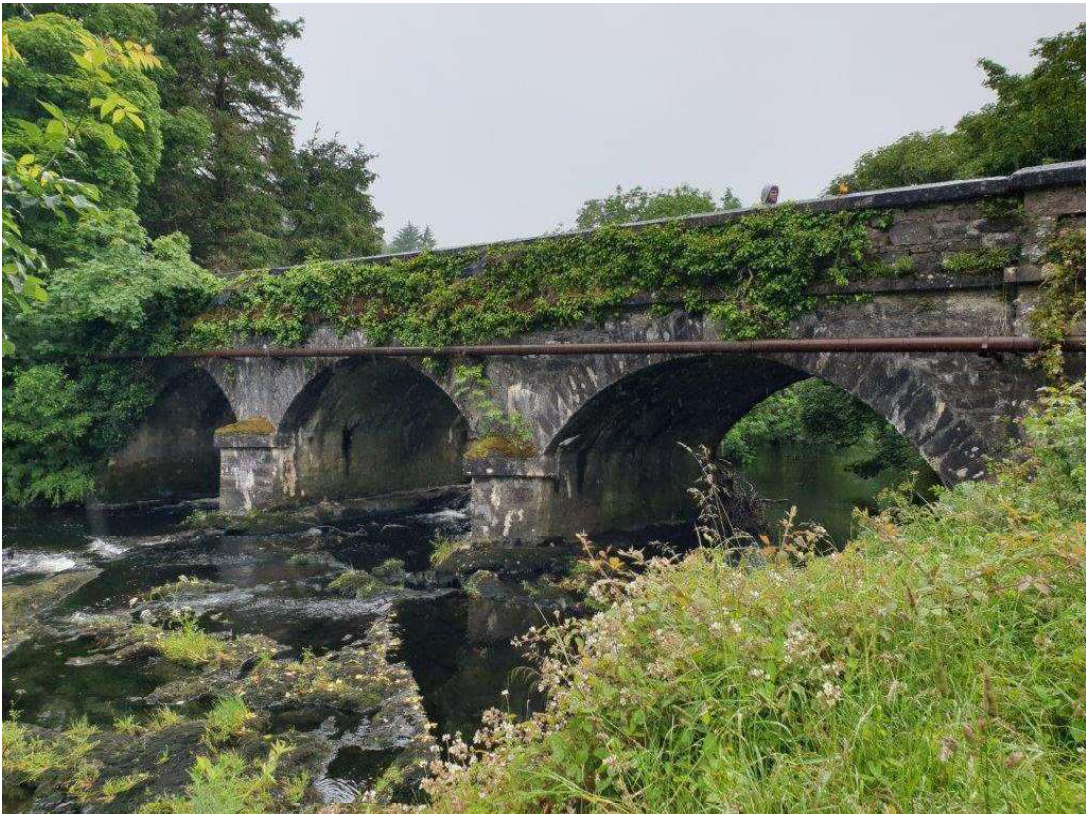
General view of the south elevation
