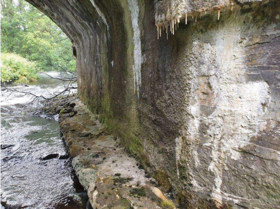
Typical pier condition
