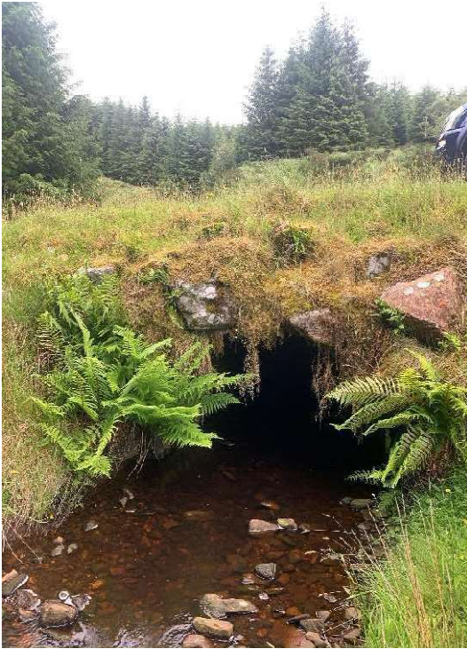
Image : 76 Box culvert crossing under road
