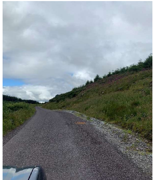
Image : 16 Joint bay on the road here with a links box and communications chambers visible.
