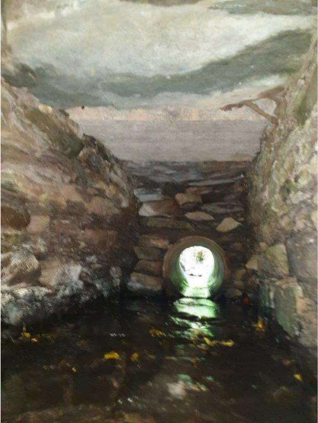
View of south span from the west
