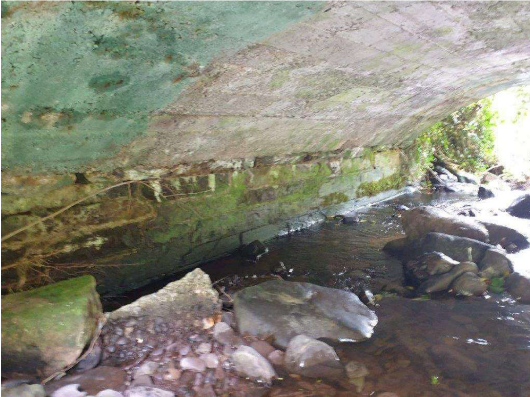
Typical condition of abutment & arch barrel
