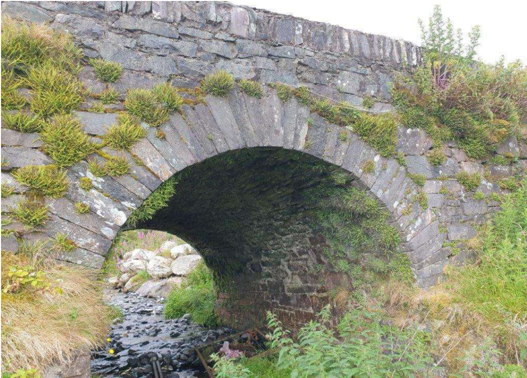
General view of the south elevation
