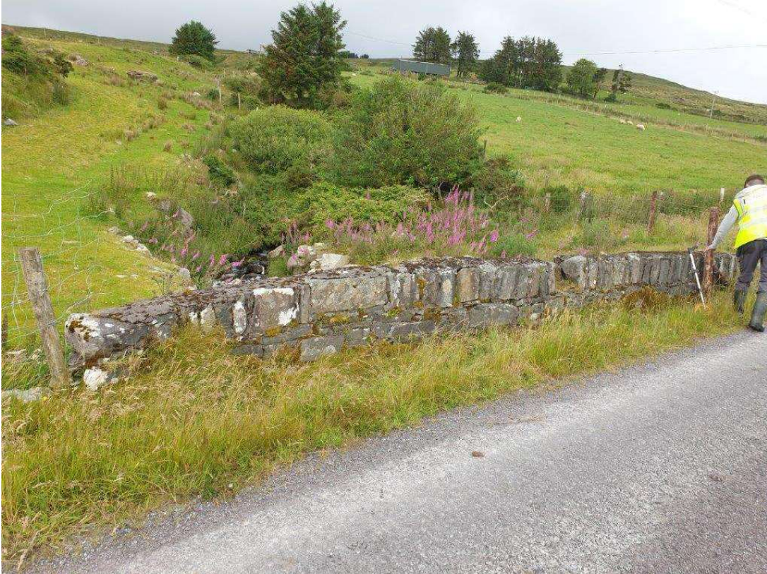
General view of the north parapet
