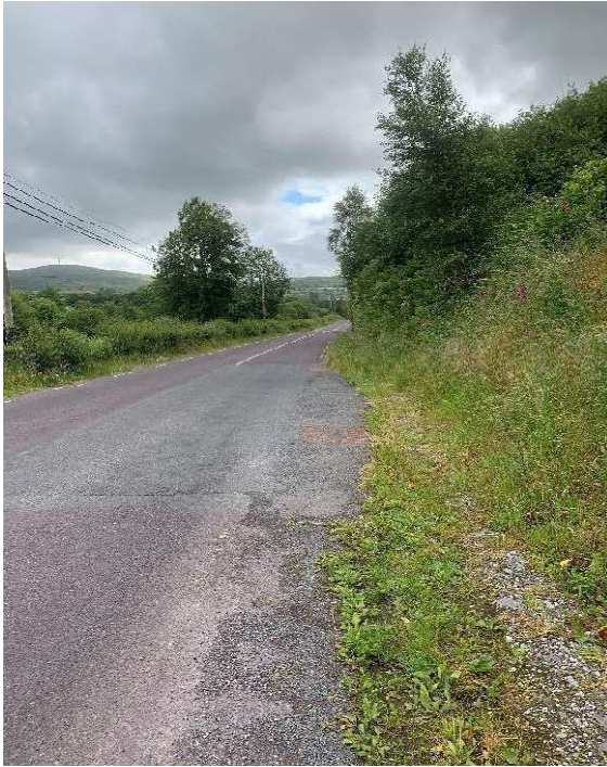
Image : 41 Joint bay on the road here with a links box and communications chambers visible.
