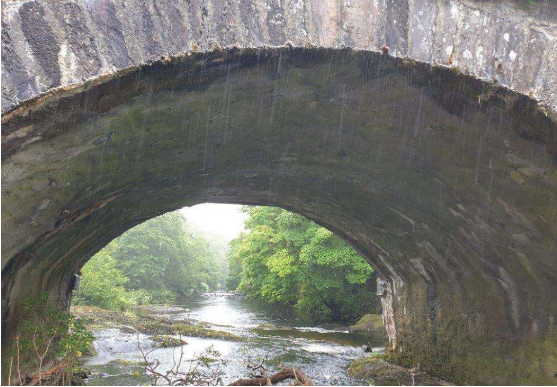
General view of the middle span, looking downstream
