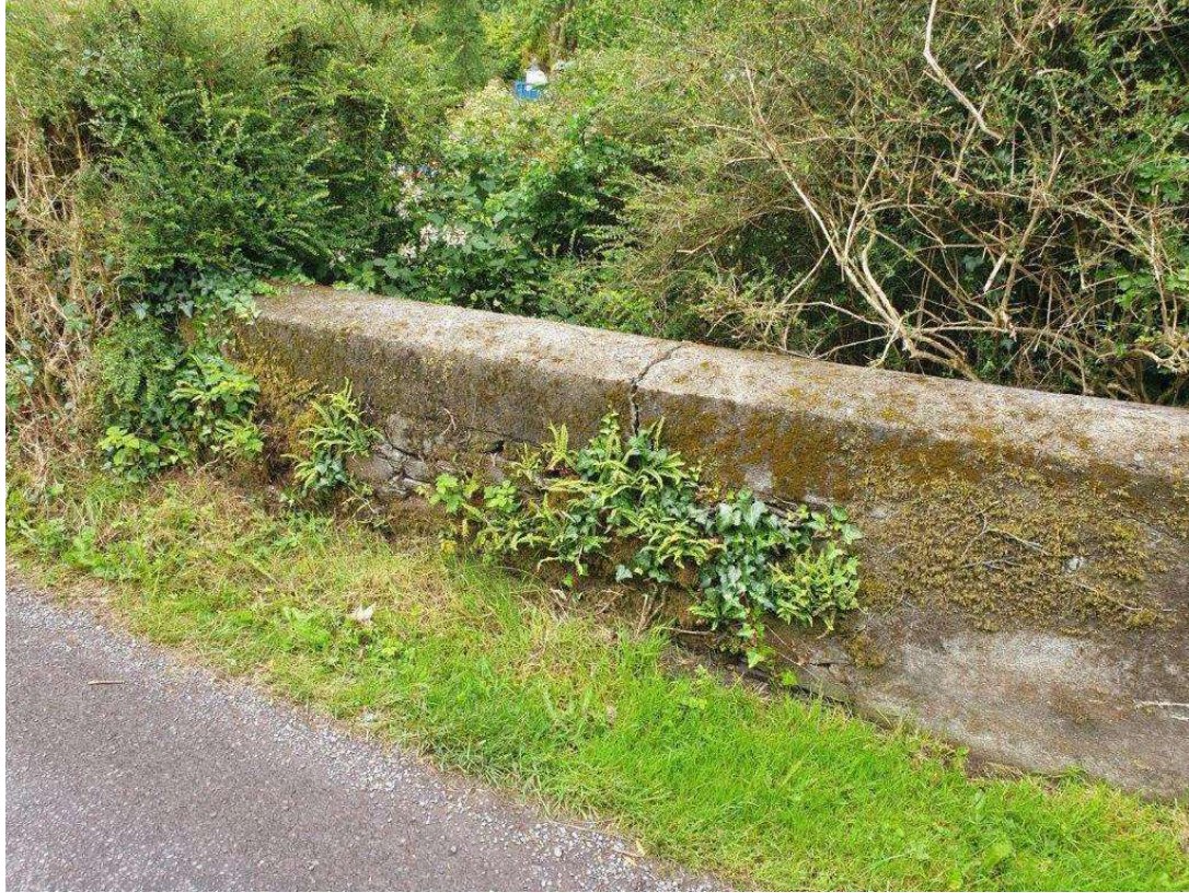
North parapet, west end
