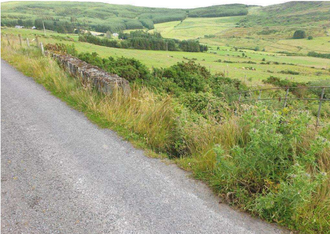
General view of the south parapet
