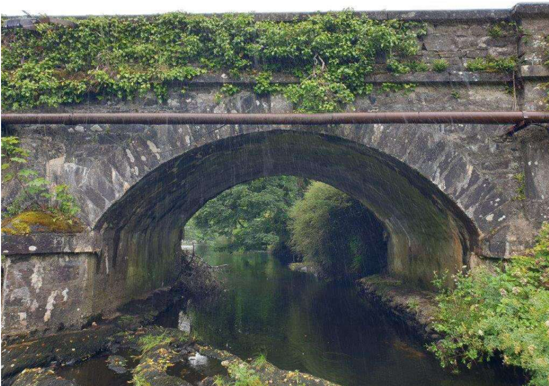
General view of the eastern span, looking upstream
