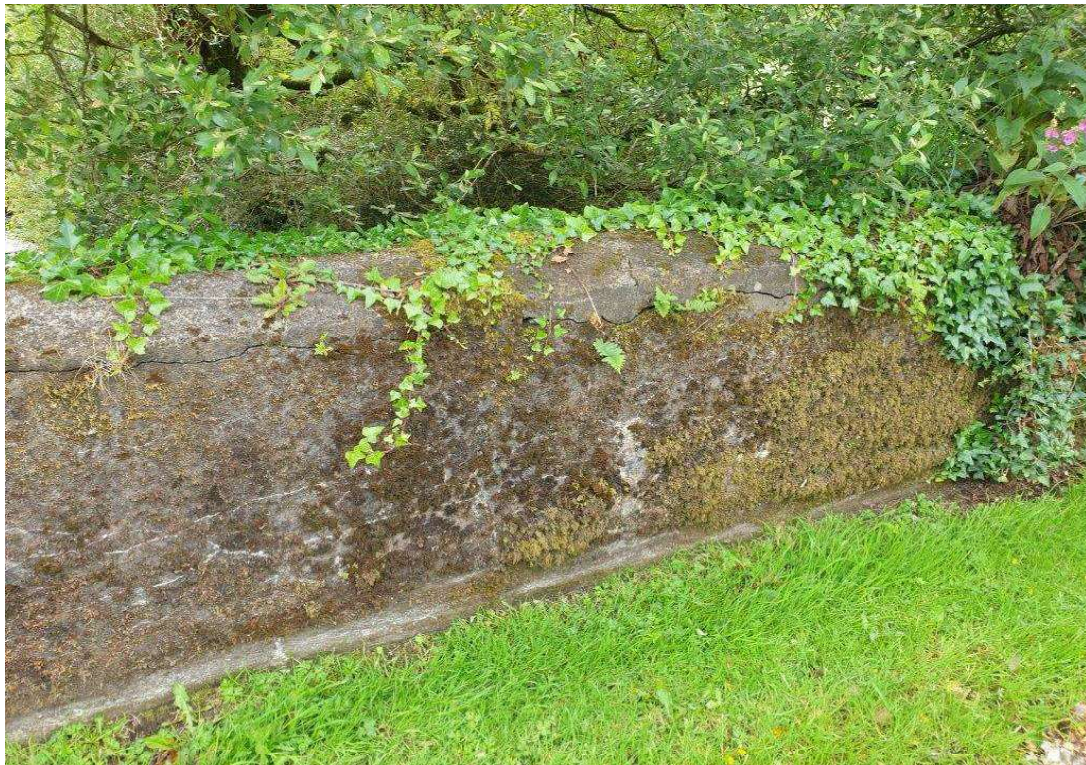
South parapet, east end
