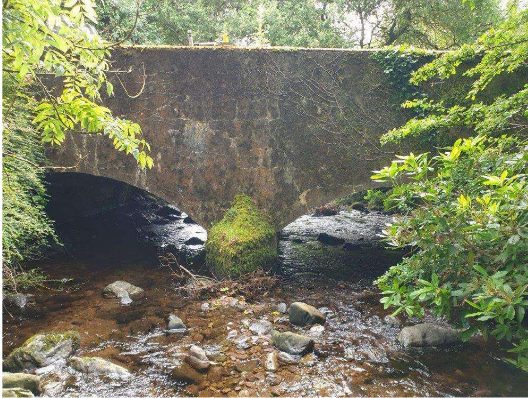
General view of the west elevation
