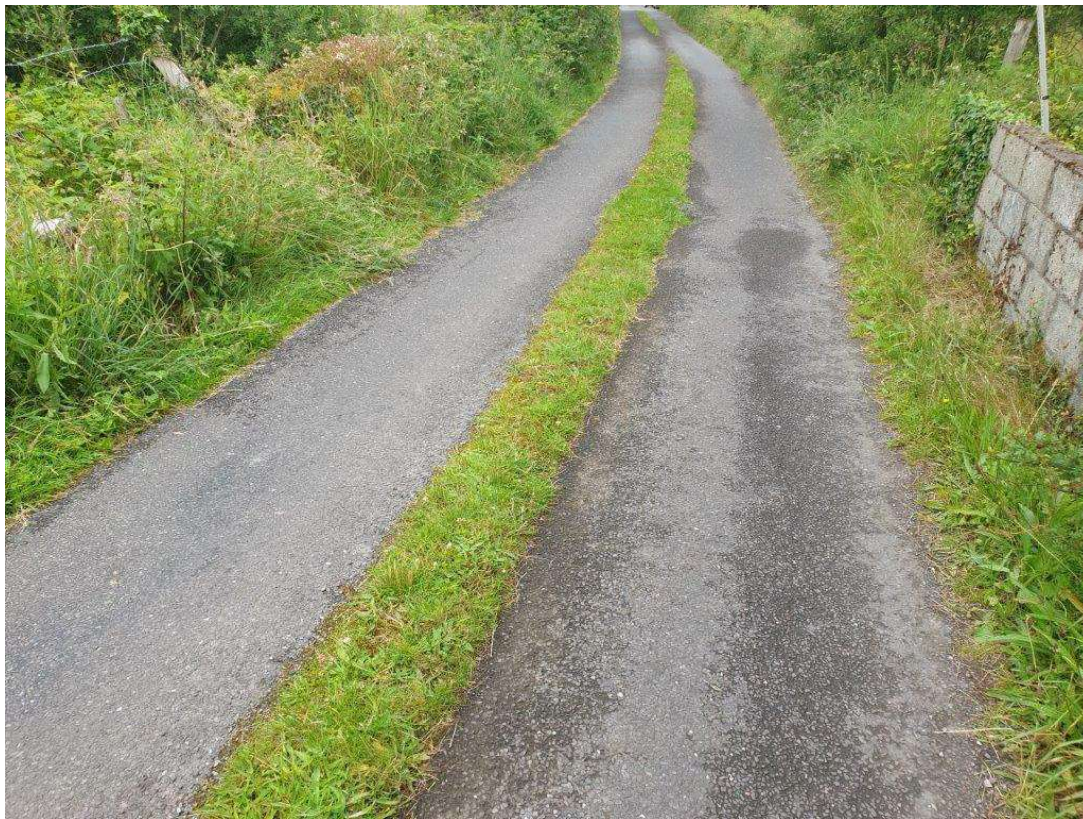
General view of bridge surface
