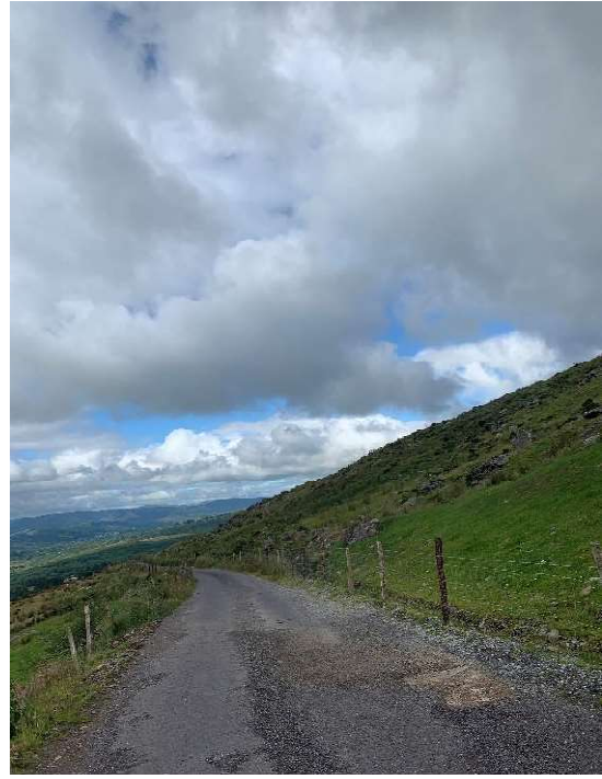
Image : 22 Joint bay visible at this location
