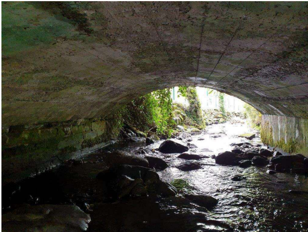
View through east arch, looking south
