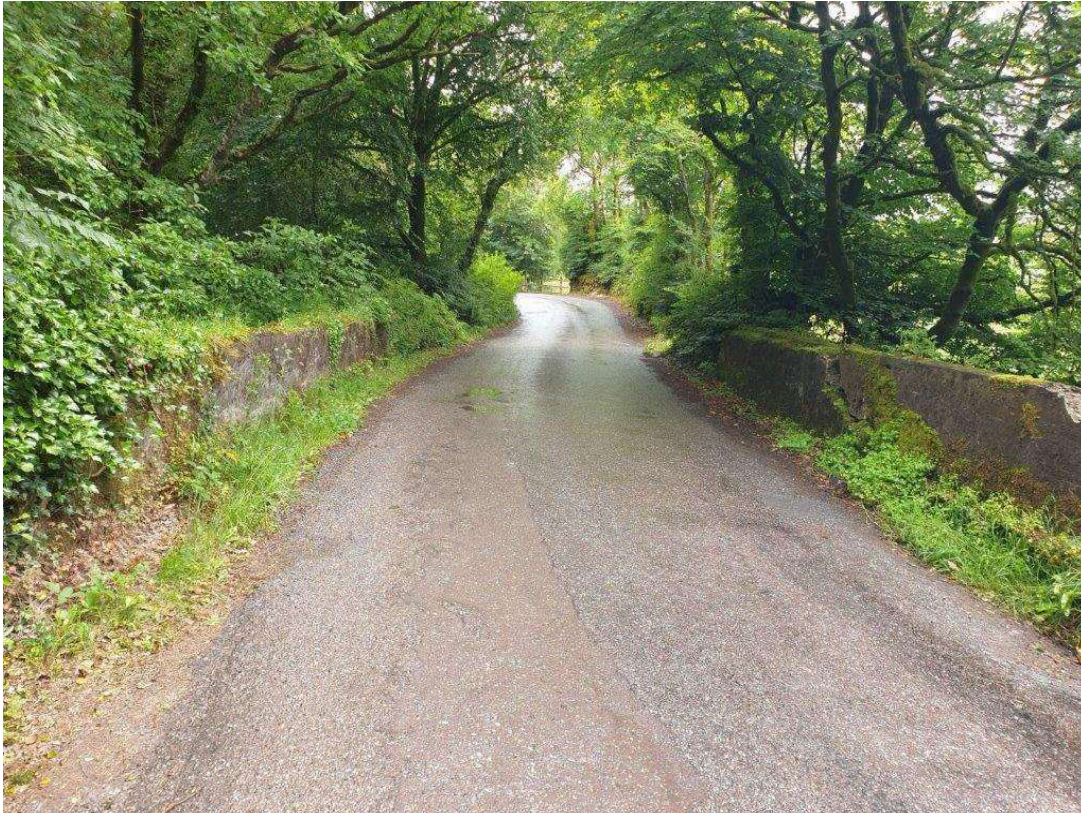
General view of the bridge surface
