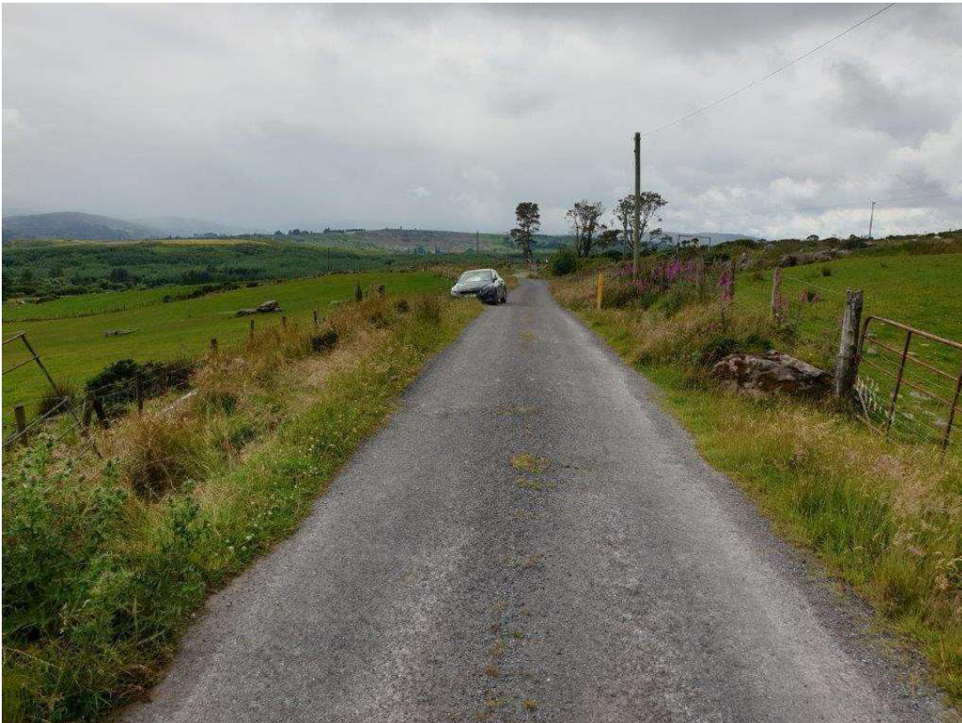
General view of the bridge surface from the east
