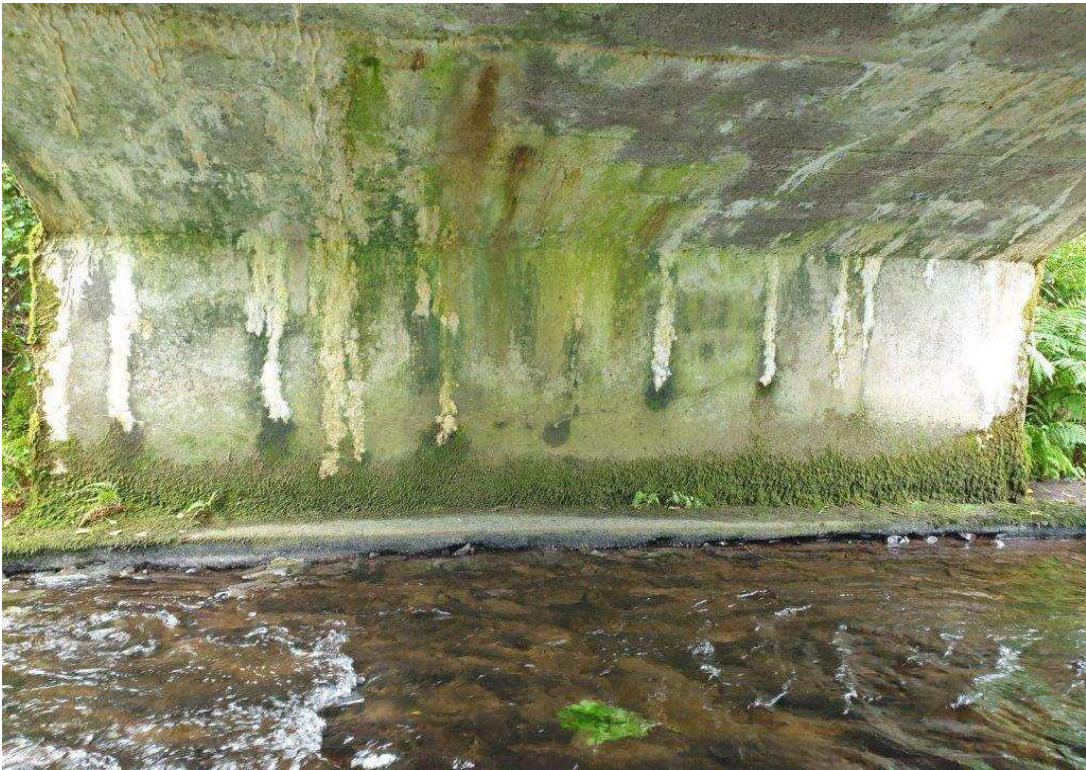
General view of the north abutment
