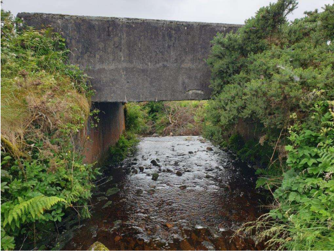
General view of east elevation, looking downstream
