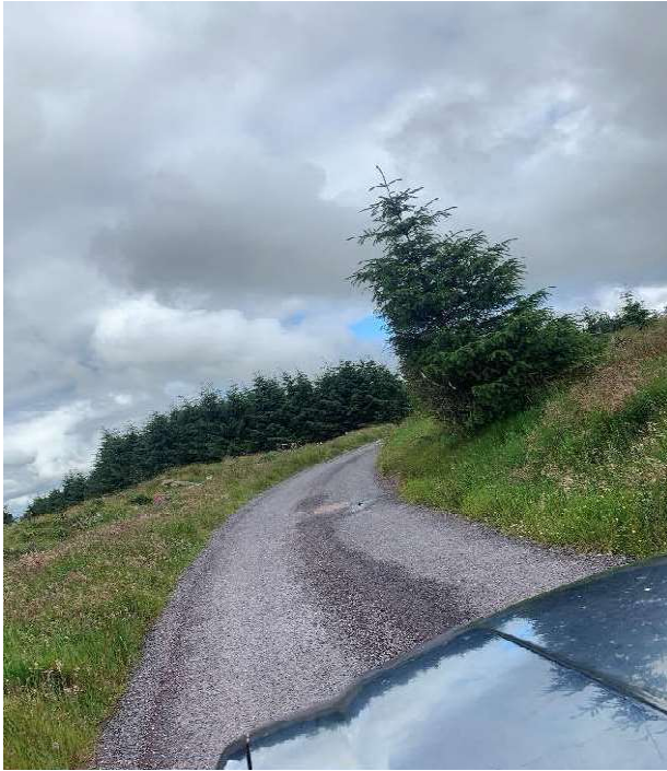
Image : 17 Joint bay located at this point
