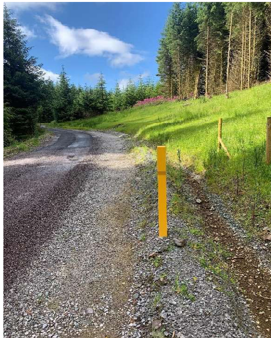
Image : 15 Ebs marker post pictured along road edge before another possible joint bay location
