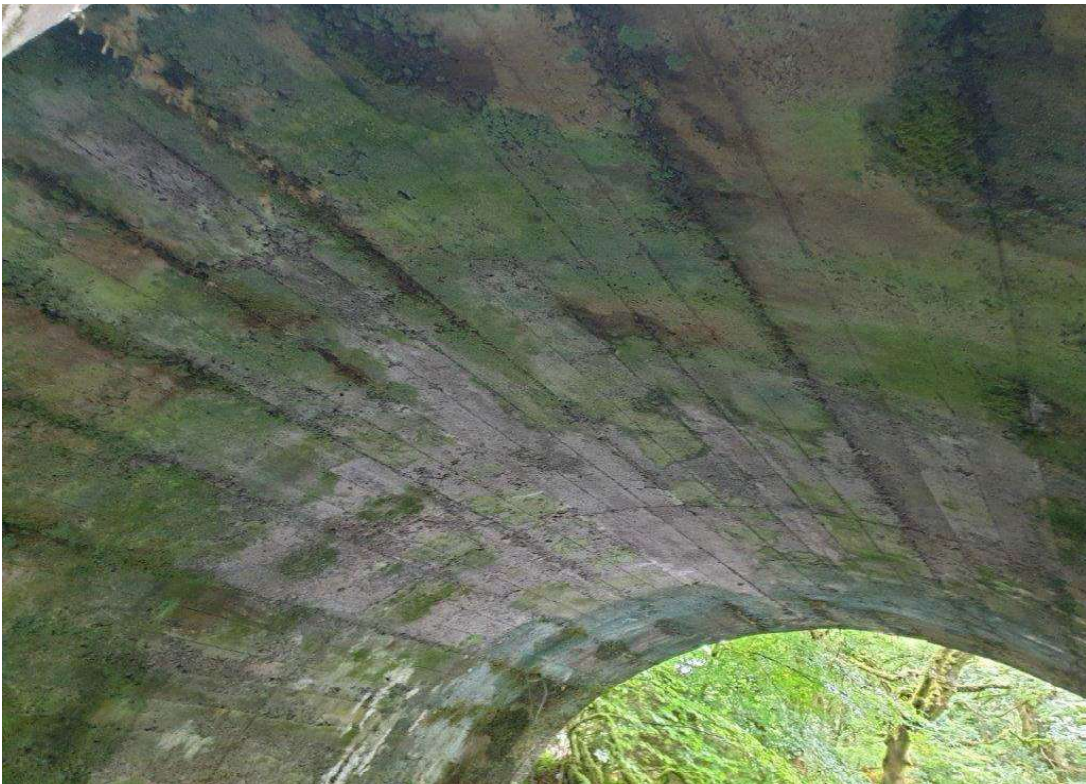
General view of the arch soffit
