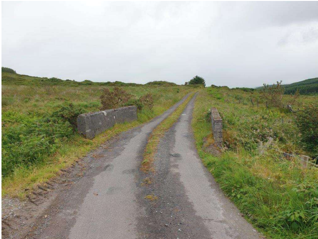
General view of the bridge surface looking south
