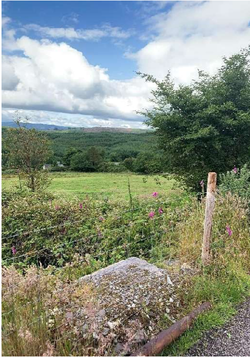
Image : 29 Storm water pipe crossing under road at this location
