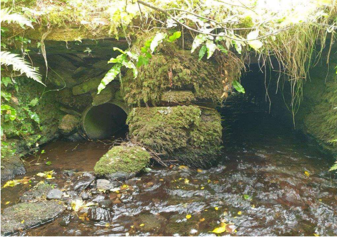
General view of the east elevation
