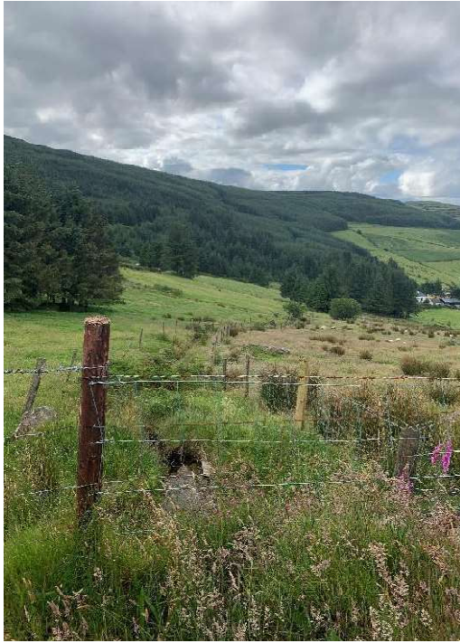
Image : 23 Storm water pipe crossing under road at this location
